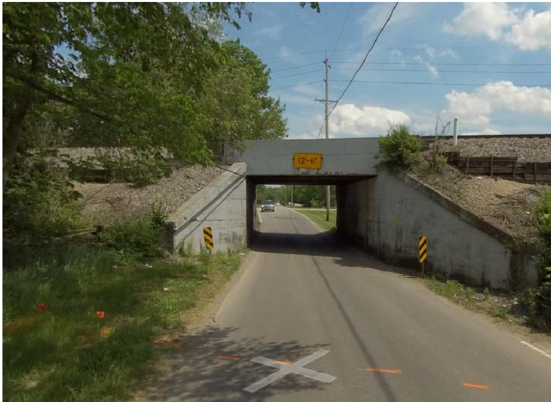
Improvements to Franklin-Trenton Road
